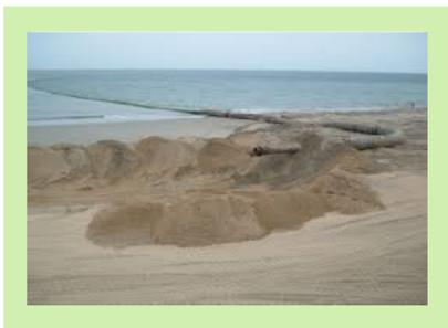
Material is dredged from the sea bed and pumped to shore along with large amounts of water. As the dredged material is pumped onto the beach the water drains away leaving the sand behind.
