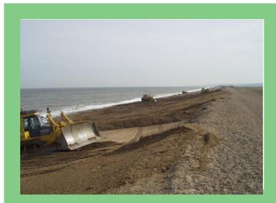
Reshaping of the beach, material is moved by machine from areas of accretion to areas where erosion has taken place.
