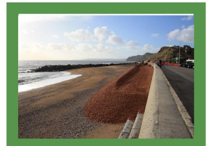
Dredge spoil from other areas or gravel / sand that has been quarried in shore can be transported to site by truck and placed where it is required.
